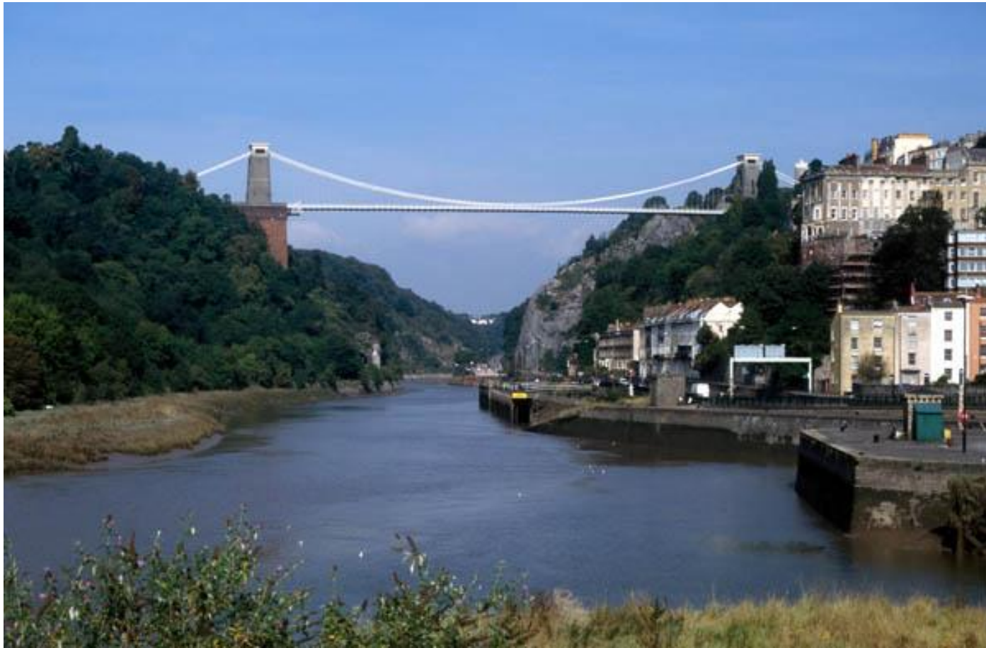
Clifton Suspension Bridge
